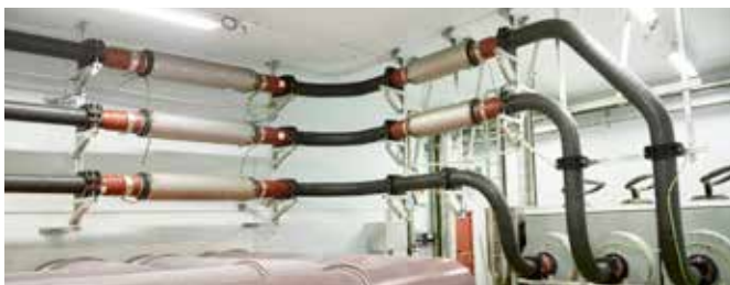
Indoor Connection 8000 A per single phase
